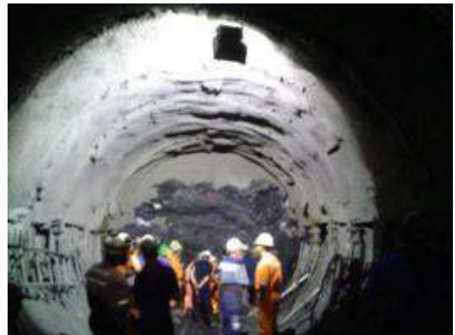
Underground excavation face view
