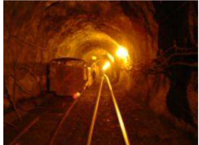
Yacambu– Quibor tunnel
