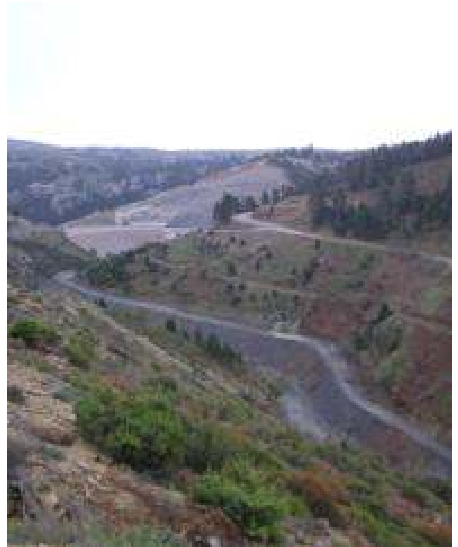
Dam, spillover and section of water flush basin view
