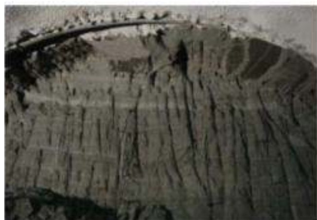
Tunnel's face – Grey Marl
