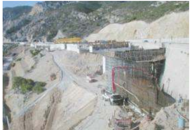
Transition part construction
