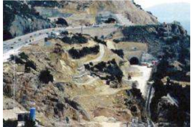
Slopes view during construction
