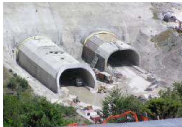
Agios Nikolaos entrance portals cut & cover structures (Egnatia Odos, section 3.3)
