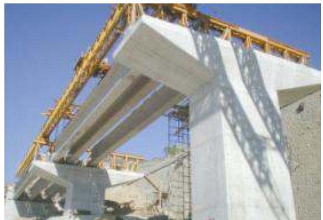
Prestressed beams construction
