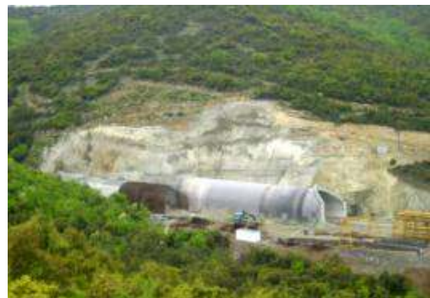
S1 tunnel entrance portal cut & cover (Egnatia Odos, section 5.2-5.3)
