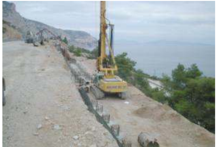
Piles construction for the foundation of a retaining wall
