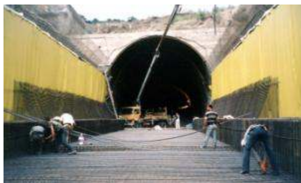
Cut & Cover base reinforcement and lateral walls construction
