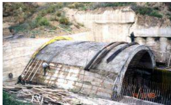
Cut & Cover crown Concreting works
