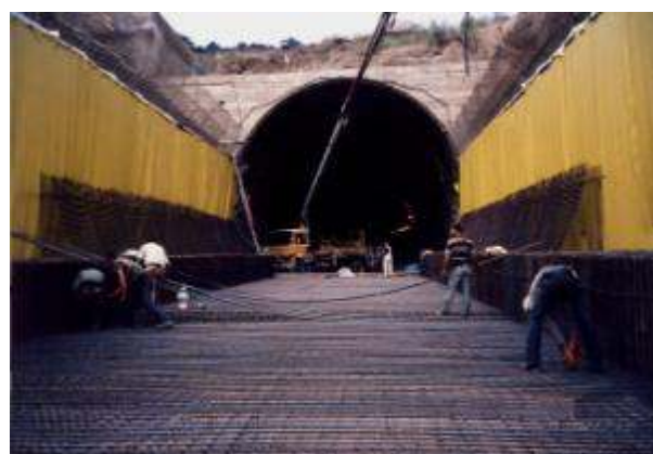
Cut & Cover structure in the exit portal
