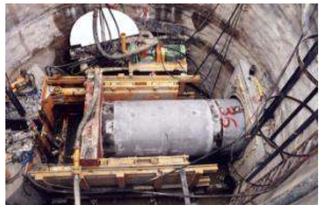
Pipe jacking entrance through the construction shaft
