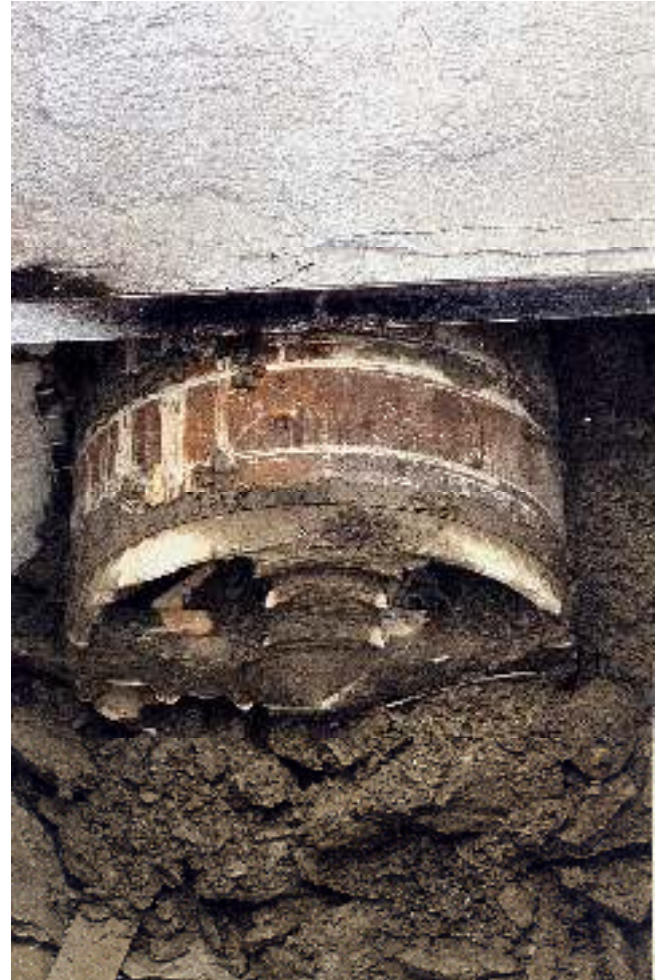
Pipe jacking breakthrough
