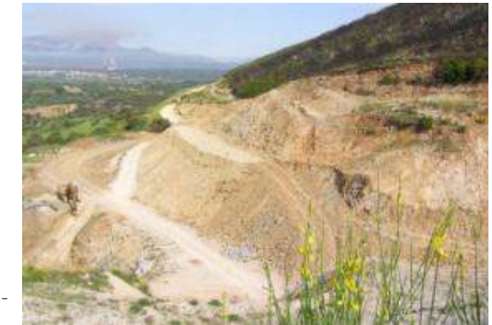
Open cut area view in Rapsomati tunnel exit
