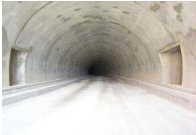
Tunnel with final lining
