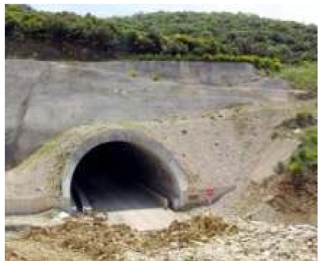
Left bore exit portal
