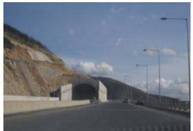
Rockfall protection area
