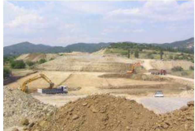
Embankment construction works
