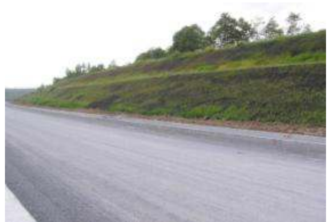
Open cut slopes view after rehabilitation
