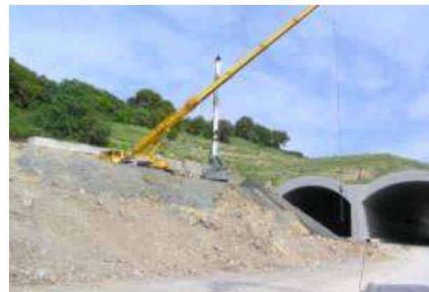
Support pile wall construction
