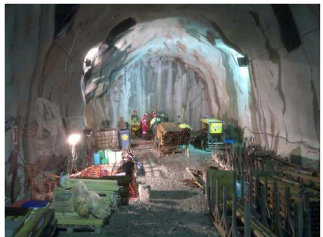
Main access tunnel during construction
