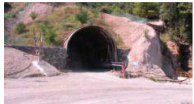
Access adit entrance +360
