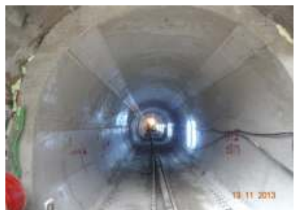
Kokkinolakkas diversion tunnel underground section
