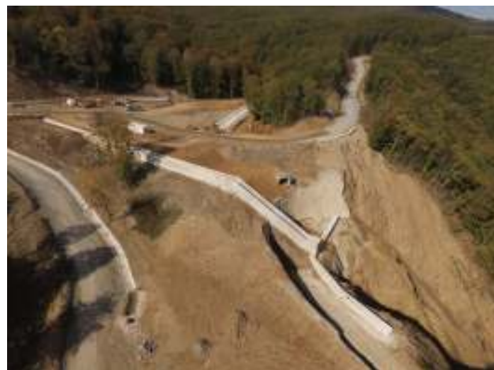
Construction works in the area of the outfall structure
