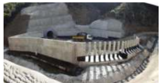
Kokkinolakkas Stream diversion tunnel & affiliated works
