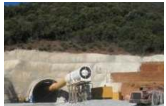
Main tunnel access works
