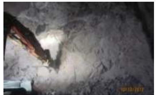
Main access & haulage Olympias tunnel
