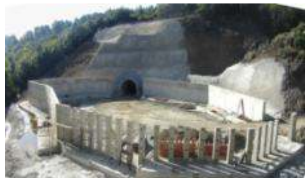
Kokkinolakkas Stream diversion tunnel & affiliated works
