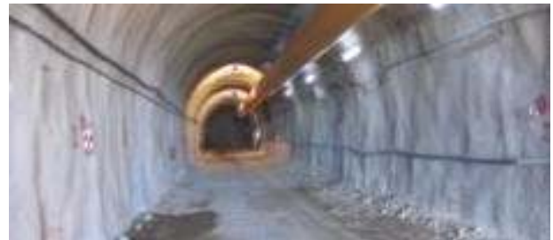
Olympias secondary access tunnel
