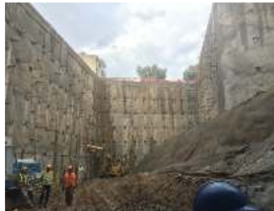
Station pit temporary support by reinforced piles and prestressed anchors
