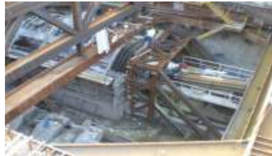
TBM installation works – false tunnel construction
