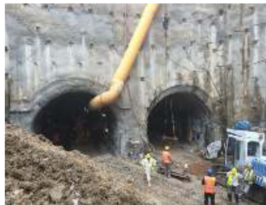
Station pit -NATM construction for the installation of the TBMs
