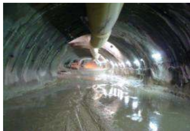
Railway tunnel during the excavation phase
