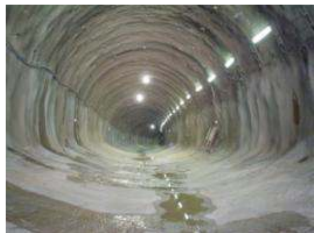
Railway tunnel, fully excavated
