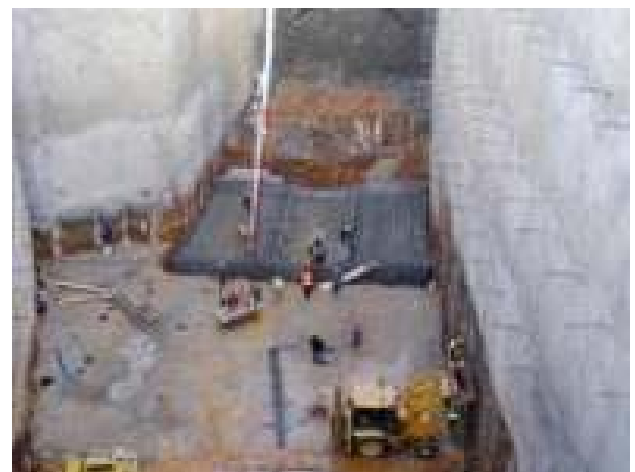
Shaft construction works
