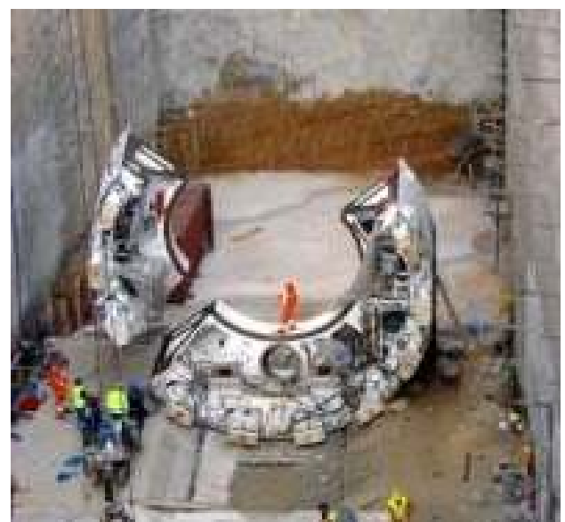
TBM assembly
