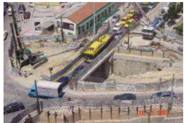
Station building pit view during construction
