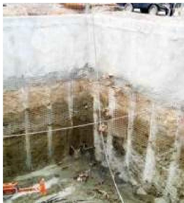
Shaft construction works
