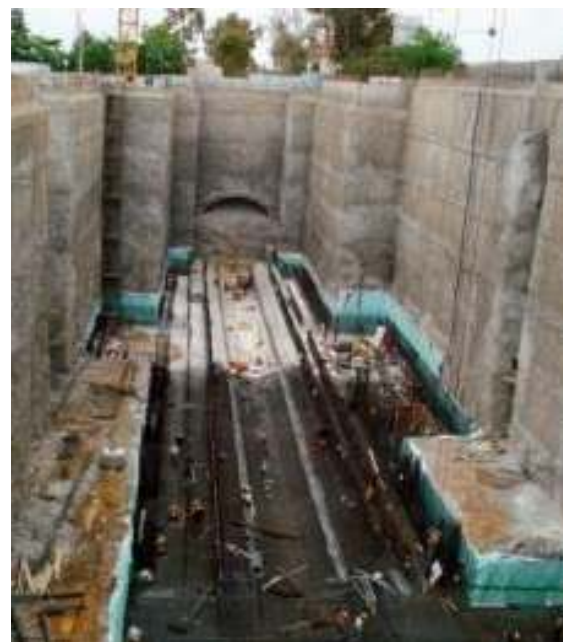
Station's construction works
