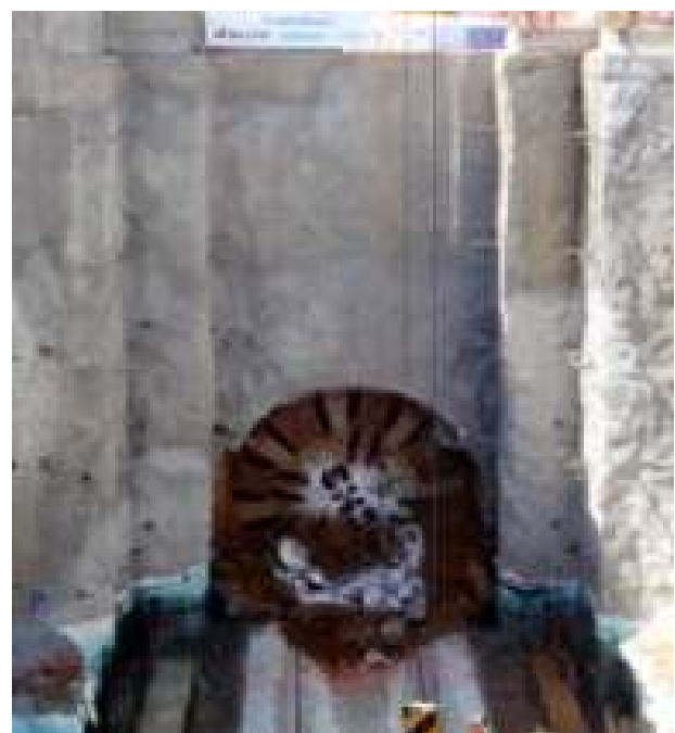
TBM's digging out at Elliniko station
