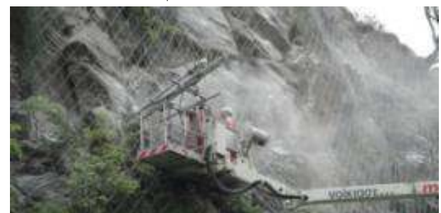
Rockfall protection barriers Installation
