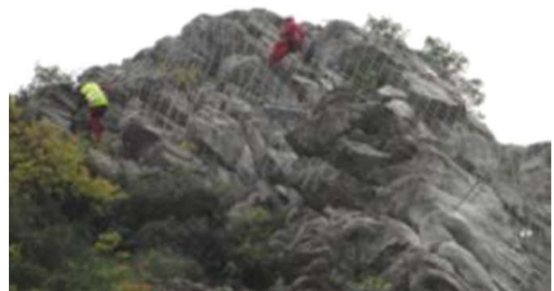
Slope stabilization systems application
