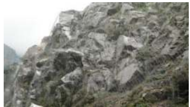
Slope stabilization system application
