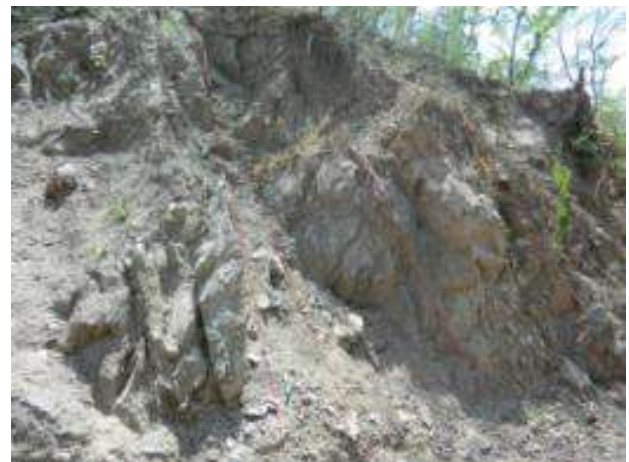
Shear zone in the area of the west portal P1 of tunnel T4
