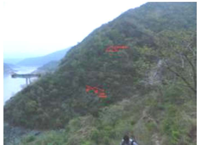
T2 tunnel – Location of portal P1
