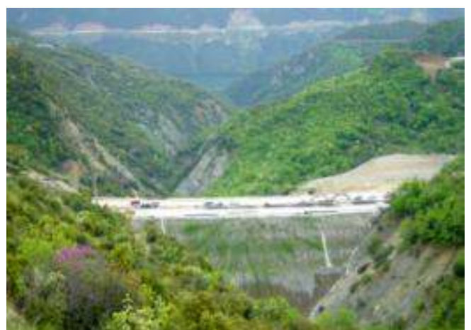
Upstream view of the embankment after the completion of works
