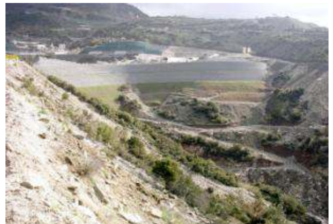
South view of the embankment
