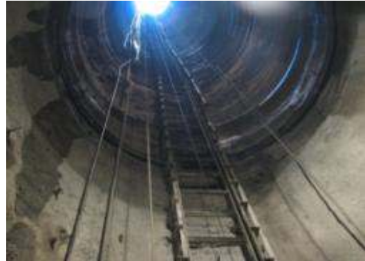
View of the smoke extraction shaft
