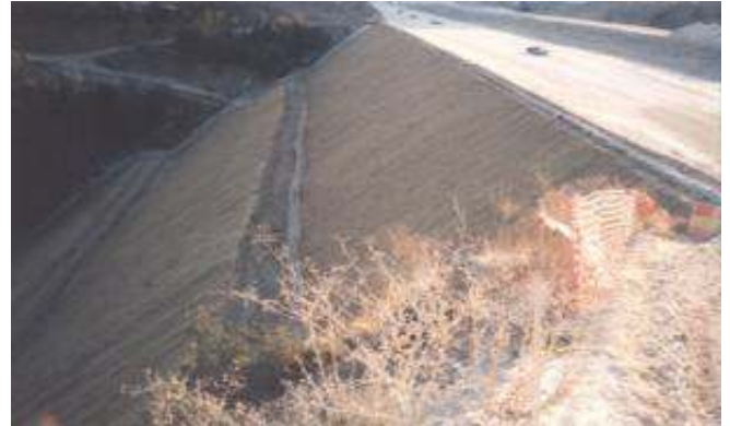
G6 rock fill embankment, maximum height 50m
