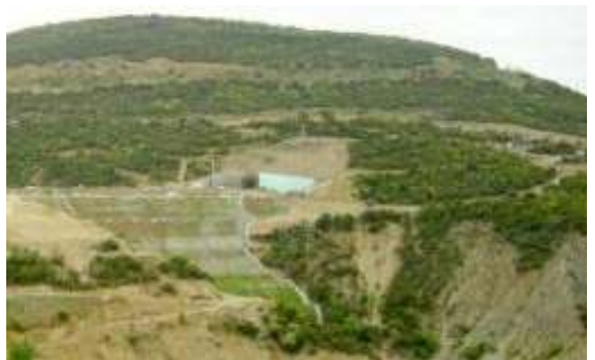
Downstream view of the embankment after the completion of works
