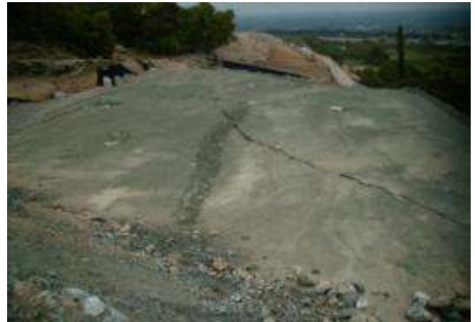
View of the embankment failure
