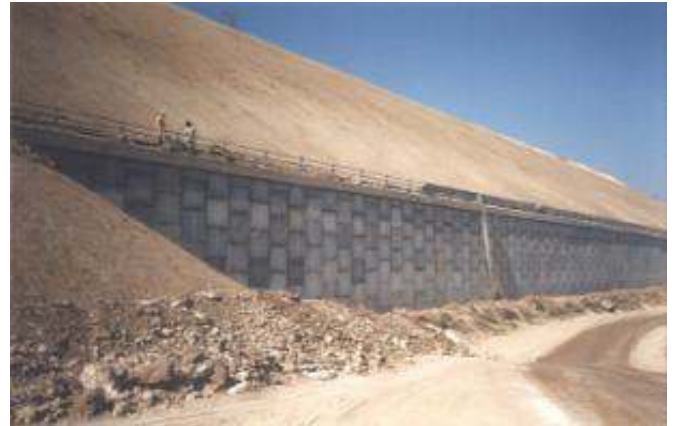
Embankment view during construction
