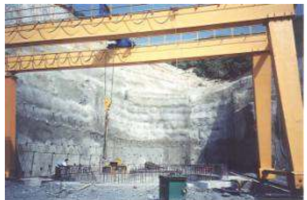
G1 bridge central pier foundation shaft retaining structure
