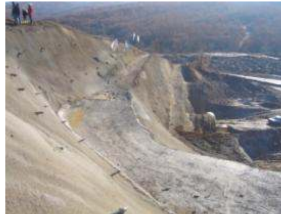
View of portals
