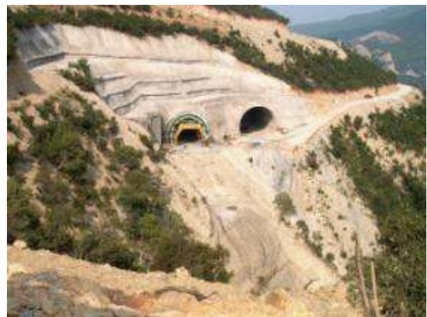
S2 exit portals
