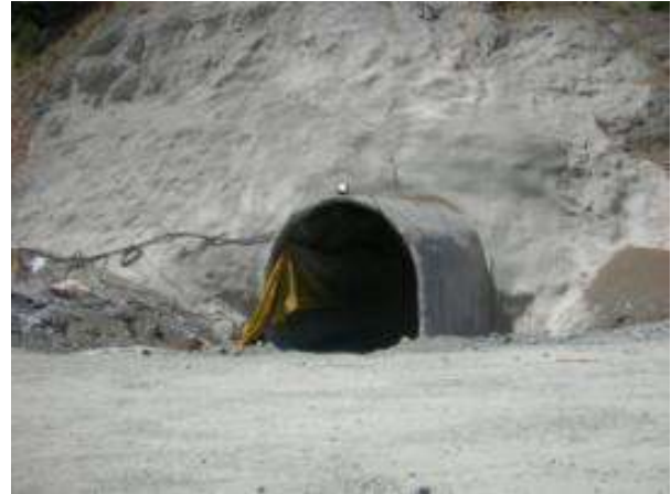
Hydraulic drainage tunnel entrance portal
