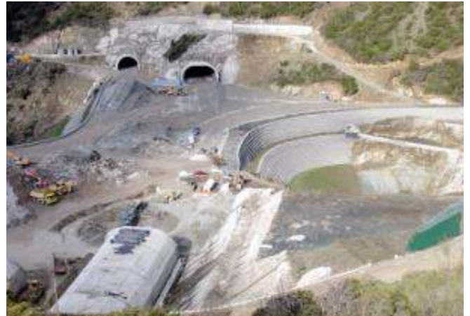
Western view of the embankment
