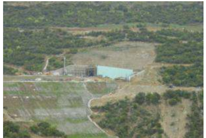
G3 reinforced embankment, maximum height 70m
