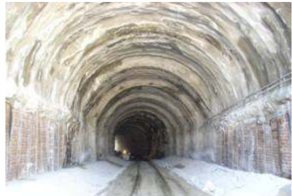
Tunnel fully excavated
