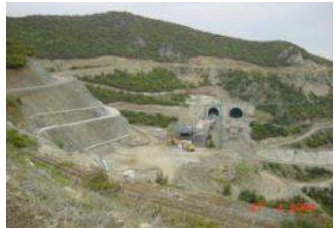
Excavated slopes in the area of the foundation of G1 bridge
