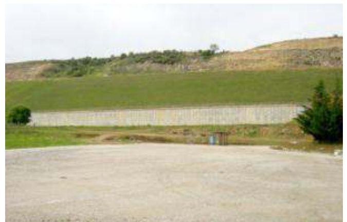
Embankment view after construction
