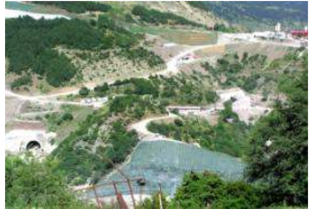
Installation of rock bolts and special grids for the slope protection against corrosion
