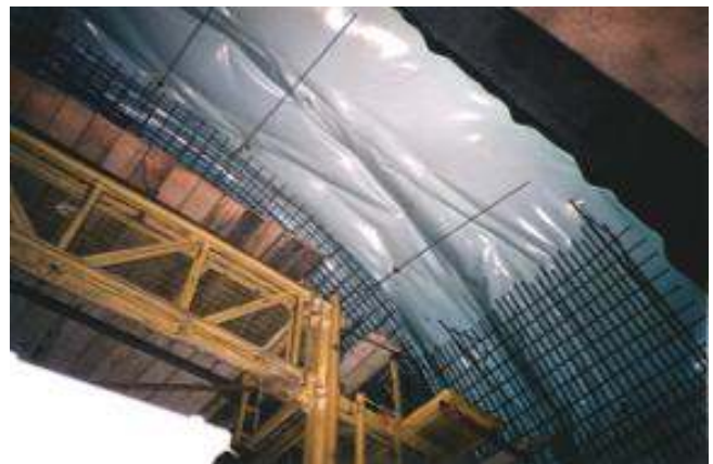
Final lining construction works
