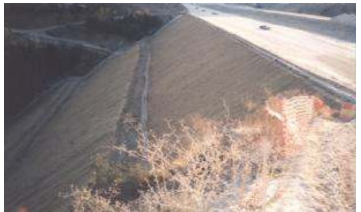
Downstream view of the embankment
