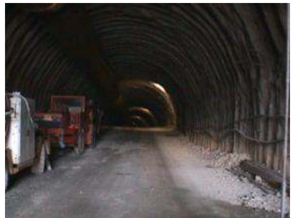
Driskos twin bore highway tunnel during a phase excavation
