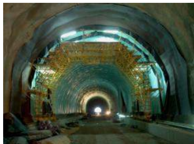
Construction of final lining in S1 tunnel
