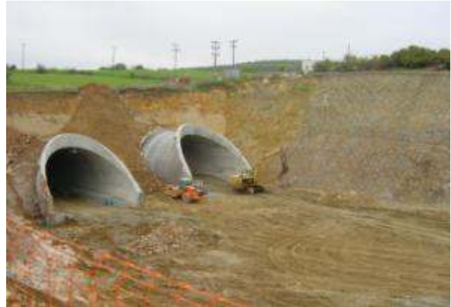
Construction works for the landscape rehabilitation of the entrance portals
