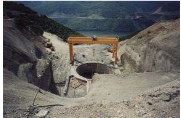
G1 Bridge central pier foundation shaft
