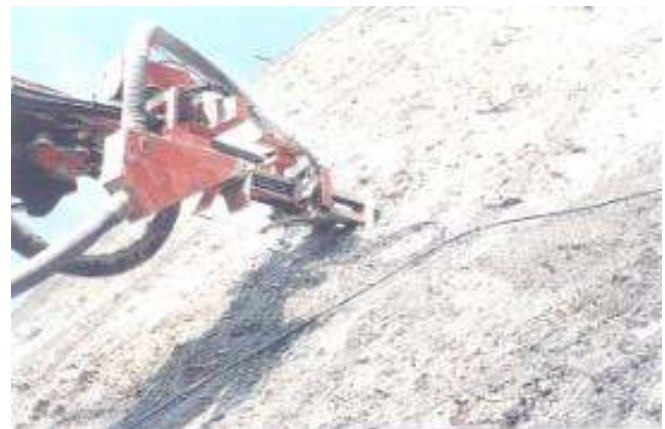
Geobrigg TECCO type grids installation works
