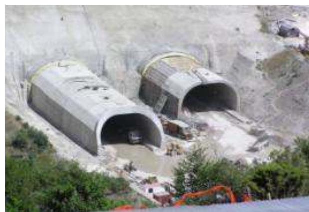
Entrance Portals Cut&Covers
