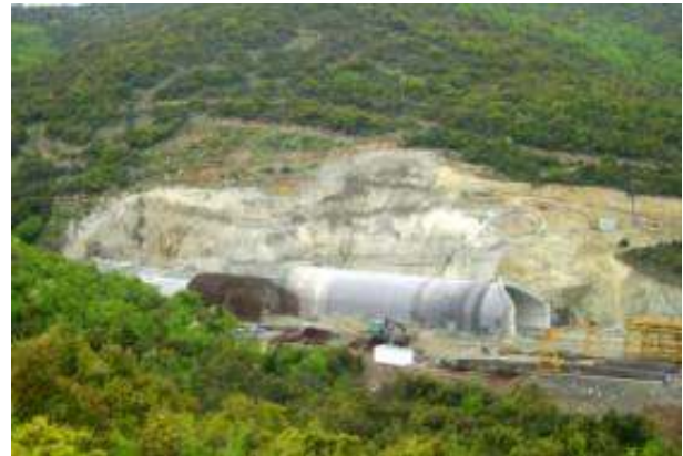
Cut & Cover entrance portals of S1 tunnel
