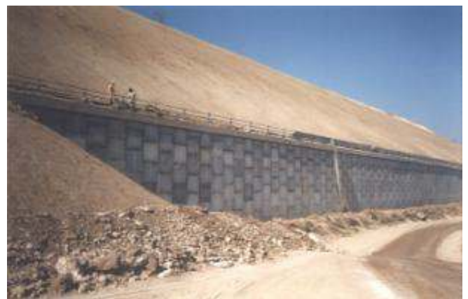
Reinforced earth embankment constructed with travertine materials and preconstructed reinforced elements, maximum height 38m
