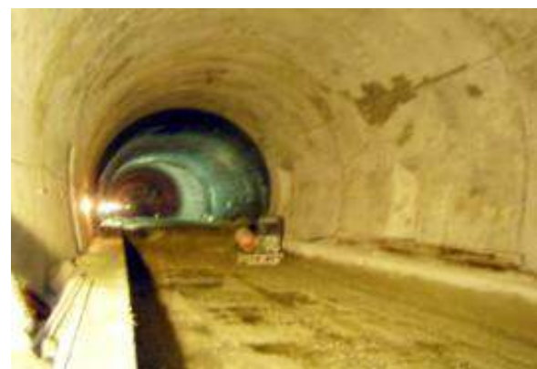
Tunnel with final lining
