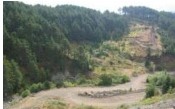
Entrance portal general view
