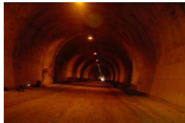
Tunnel with final lining
