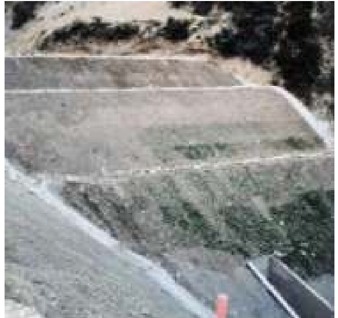
View of the embankment during the construction phase
