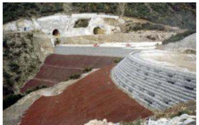
Reinforced earth in the upper slope
