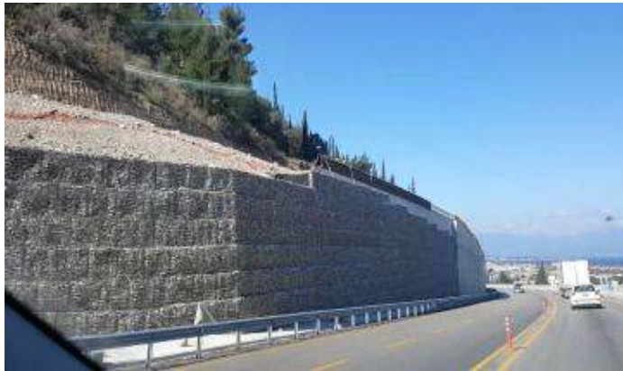
Mechanically stabilized earth-wall
