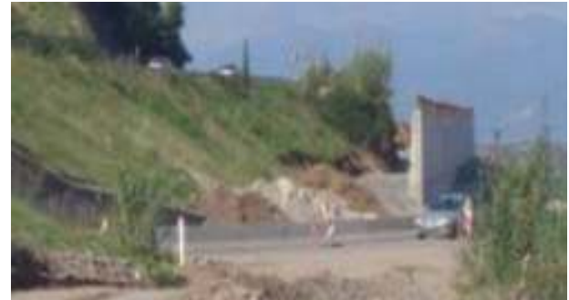
Retaining wall general view
