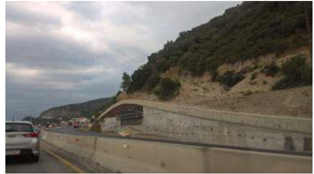
Pilewall retaining system with prestressed anchors
