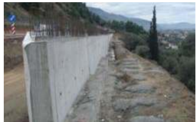
Retaining wall construction
