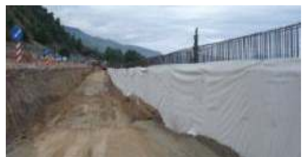
Embankment construction behind the retaining wall
