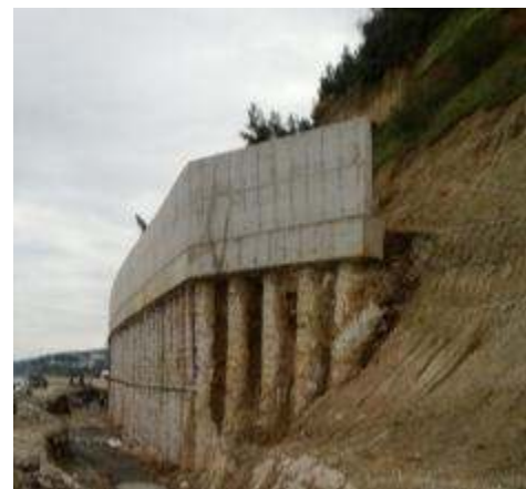
Composite retaining system with prestressed anchors
