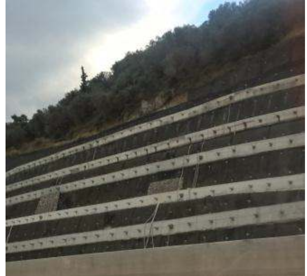
Open cut with prestressed anchors
