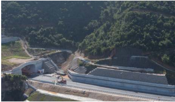
Retaining pilewall and surface protection with gabions
