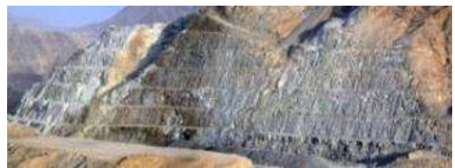
Existing rocky cut slopes
