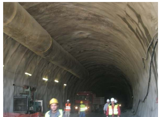
Tunnel's excavation face and underground stretch with the primary support measures
