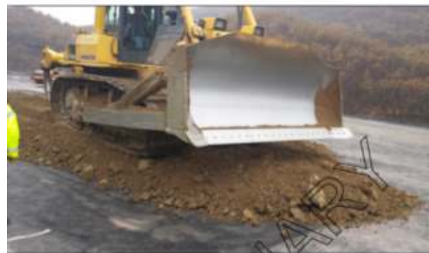
Placement and leveling of fill material
