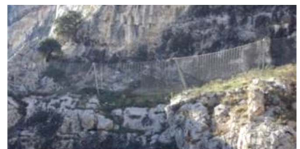
Rockfall protection barriers at the north right and left gorge portals of tunnel T1
