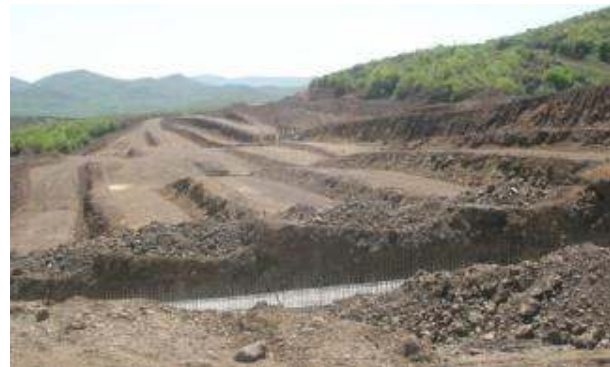
Modulation of embankments' anchoring benches
