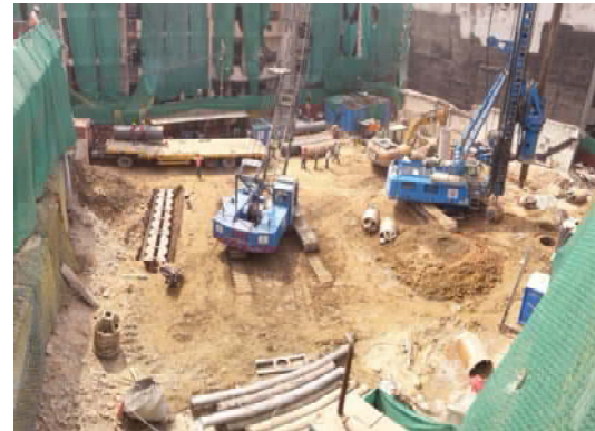
Pile construction – Rescue Shaft
