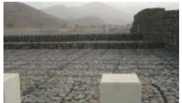
Gabion drop structure view
