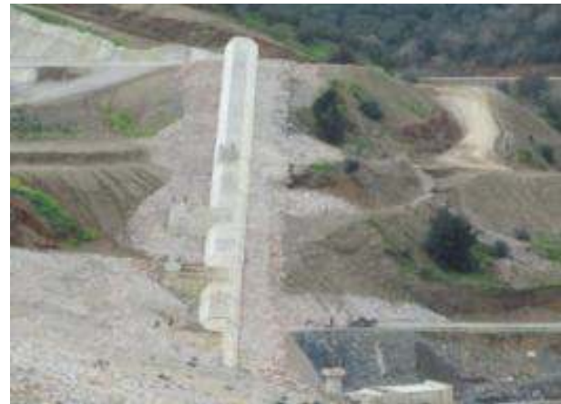
Water intake structure view
