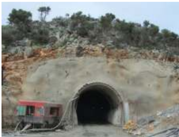
Tunnel S2 Entrance
