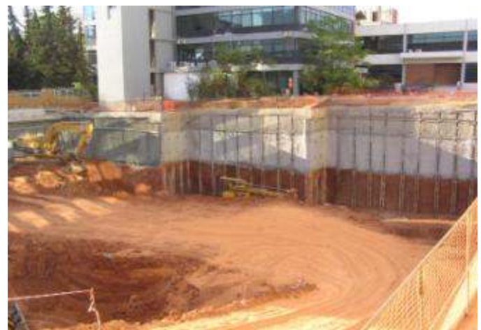
NE construction view
