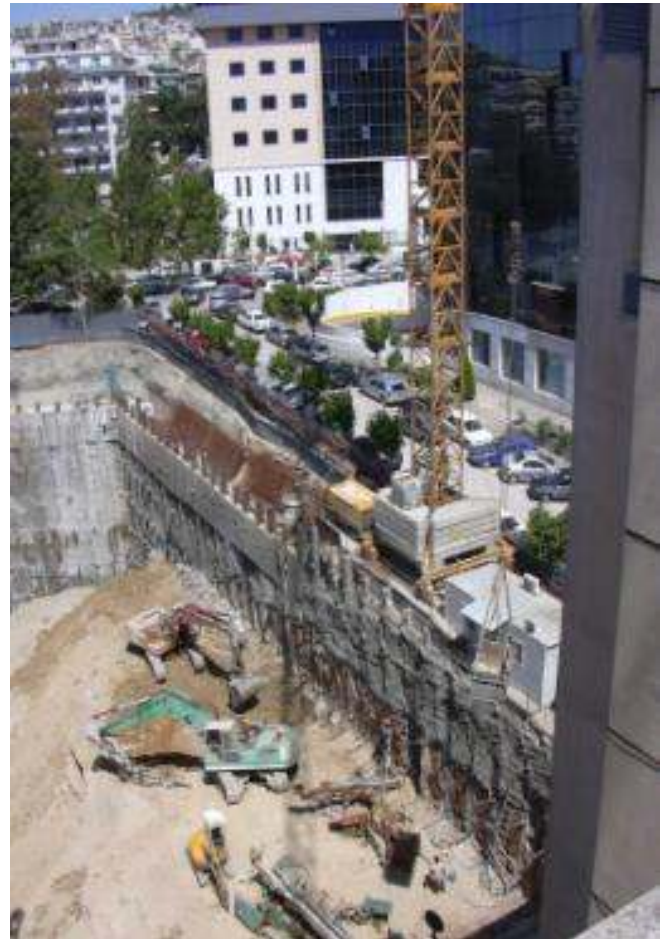
Construction site NE view
