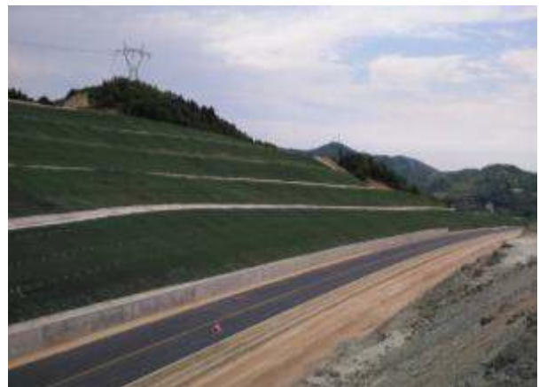
Already constructed sections of the roadway open cut
