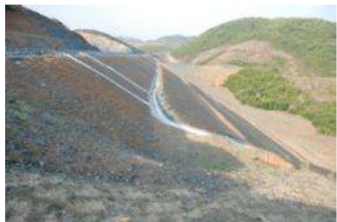
Highway embankment slopes view
