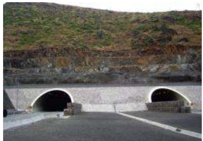
Existing Thirra tunnel
