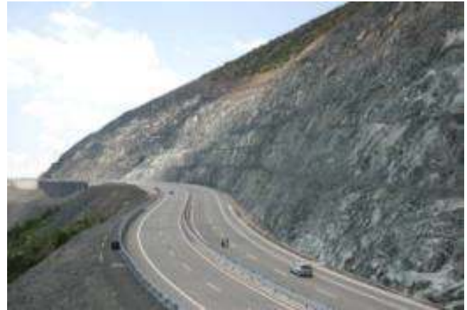
Highway cut slopes view
