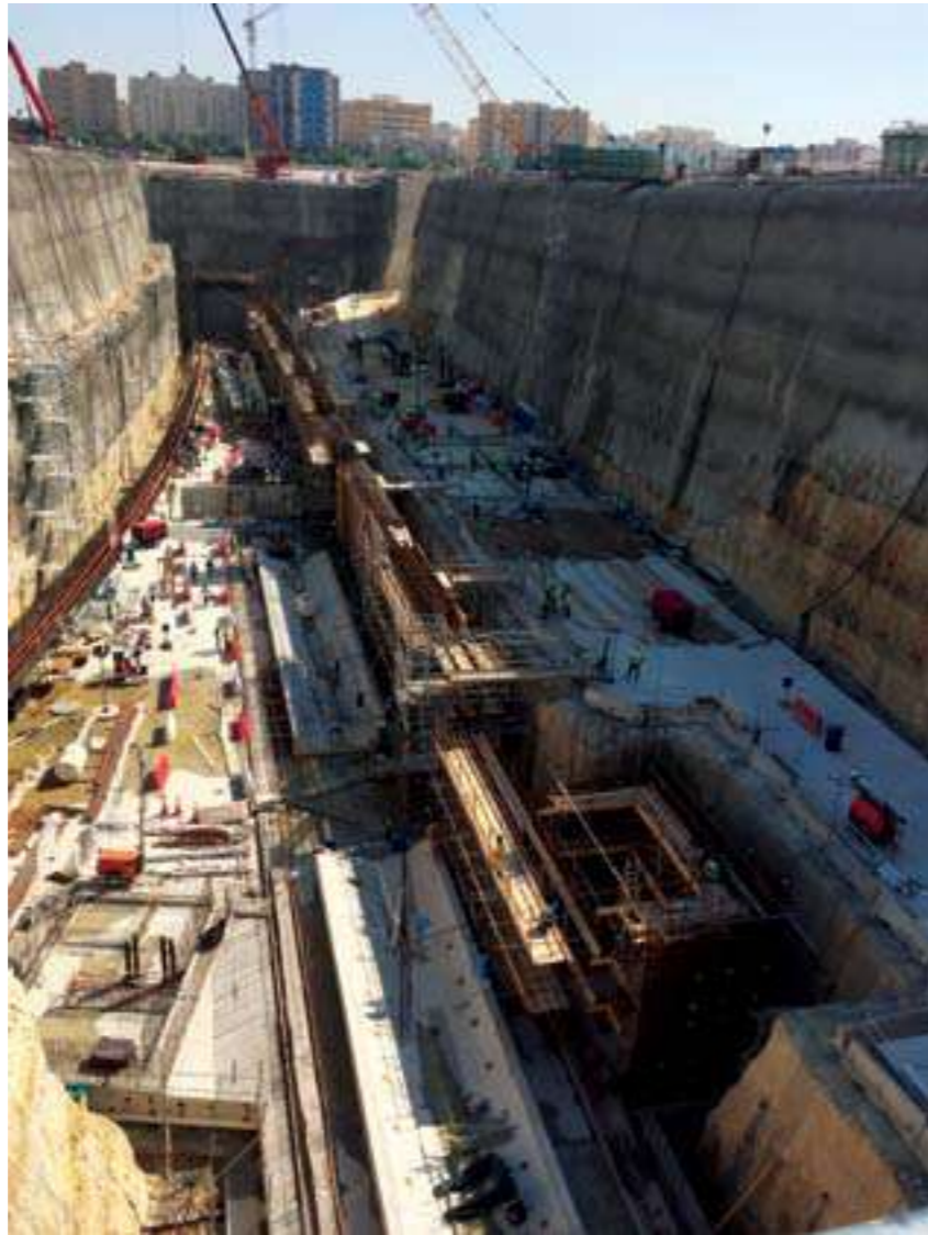
Above: Construction work in Doha
