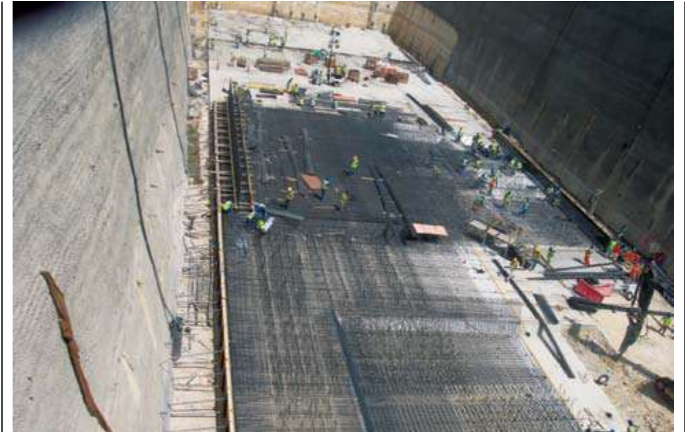
Above: Work for new metro lines being built in Doha
