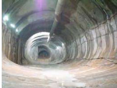
Photo 2: Final excavation geometry of the station tunnel.
