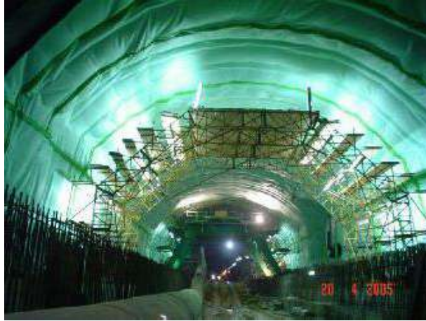
Photo 10: Installation of waterproofing membrane in the crown of the station tunnel.
