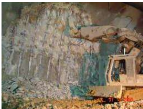
Photo 4: Demolition of station tunnel's shotcrete shell.
