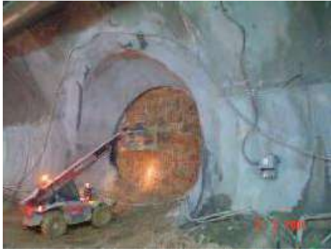
Photo 6: Protective measures on final excavation face of part 1.
