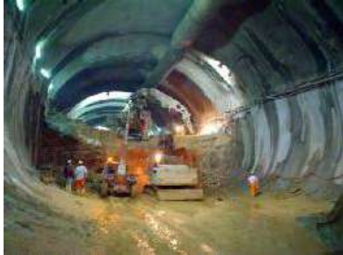
Photo 1: Bench excavation of the station tunnel.
