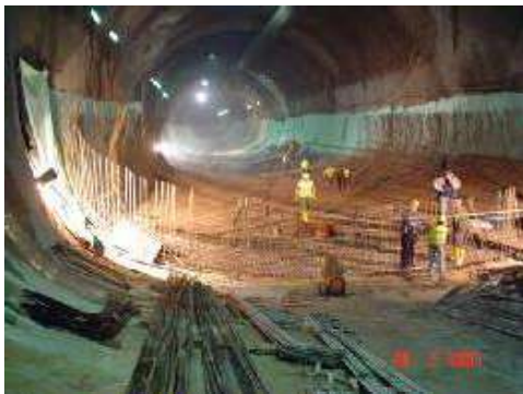
Photo 8: Installation of steel reinforcement in the final invert of the station tunnel.
