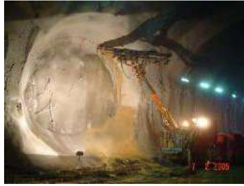
Photo 7: Installation of final row of self drilling spiles for future excavation of part 2. Gallery's face is secured with fibreglass bolts and 30cm shotcrete.
