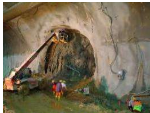
Photo 5: Installation of the second steel set HEB140.
