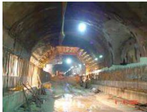
Photo 9: Completed final invert of station tunnel.
