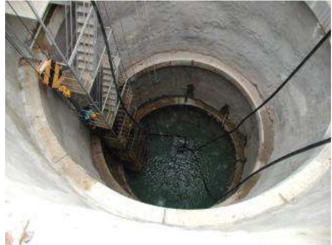
Figure 4. Shaft during pump-out test.
