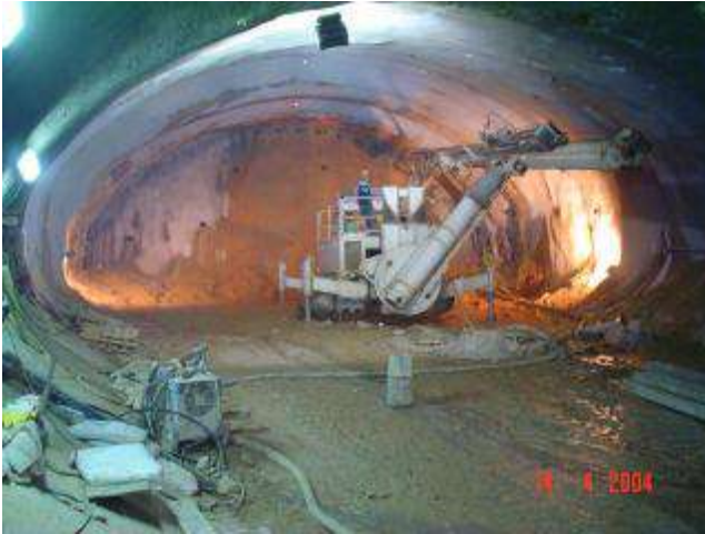
Figure 5. Installation of the forepoling tubes at the top heading of the Station tunnel.
