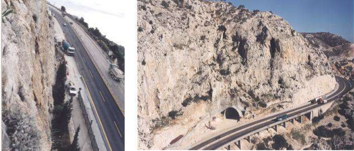
Figure 2 Extremely steep morphology in the area of the tunnels of Kakia Skala.
