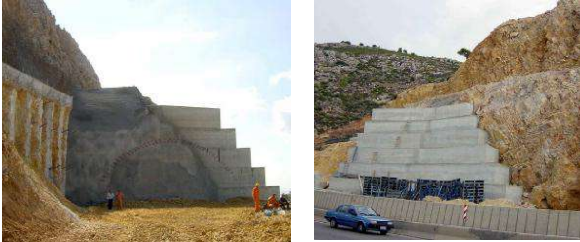
Figure 4 Reinforced concrete structure in west portal of left bore of AS1.
