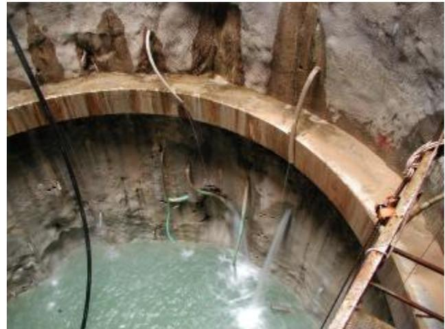
Figure 5. Water inflow from drainage holes in the shaft.
