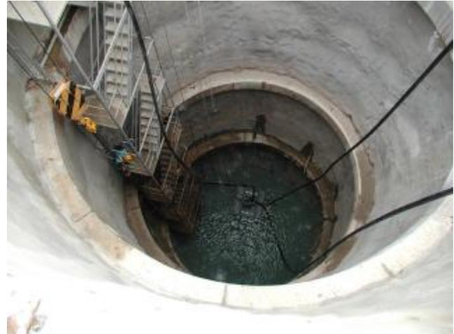
Figure 4. Shaft during pump-out test.
