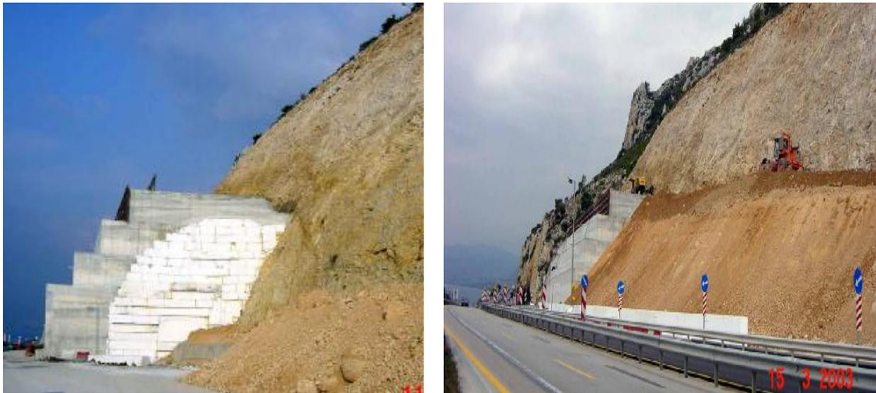
Figure 3 Reinforced concrete structure in east portal of right bore of AS1 with polysterine.
