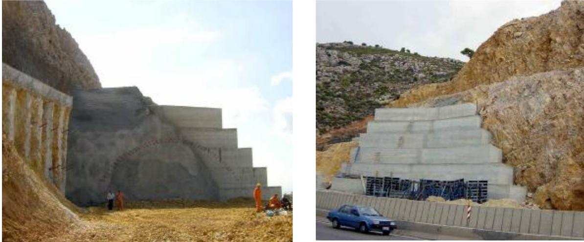
Figure 4 Reinforced concrete structure in west portal of left bore of AS1.
