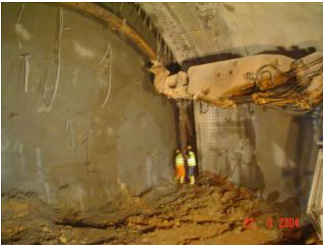
Figure 6. Top heading excavation of the Station tunnel. Installation of the HEB 180 steel arches.
