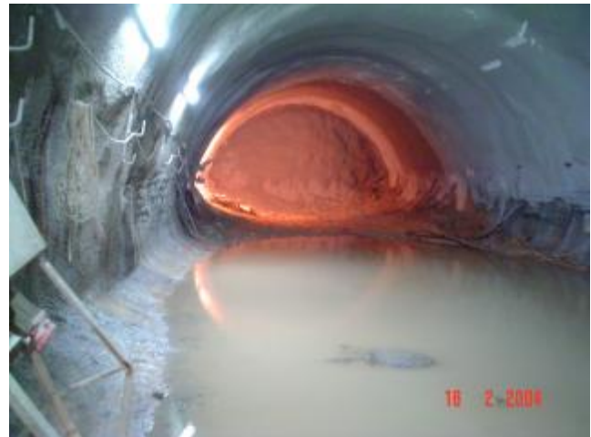
Figure 4. Top heading construction of the transition section of the running tunnel.
